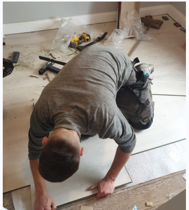
Floor getting fitted at bedroom refurbishment for 3 young sisters.
