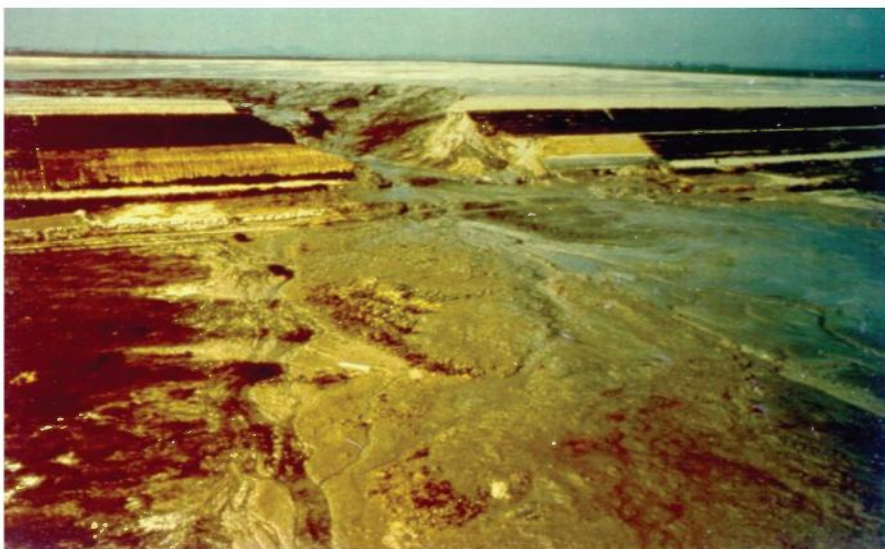
Figure 3: Failure of the Boliden lead-zinc tailings dam in 1998
