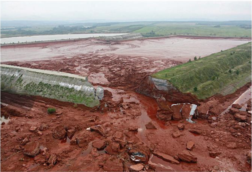
Figure 2: Failure of Hungarian Dam
