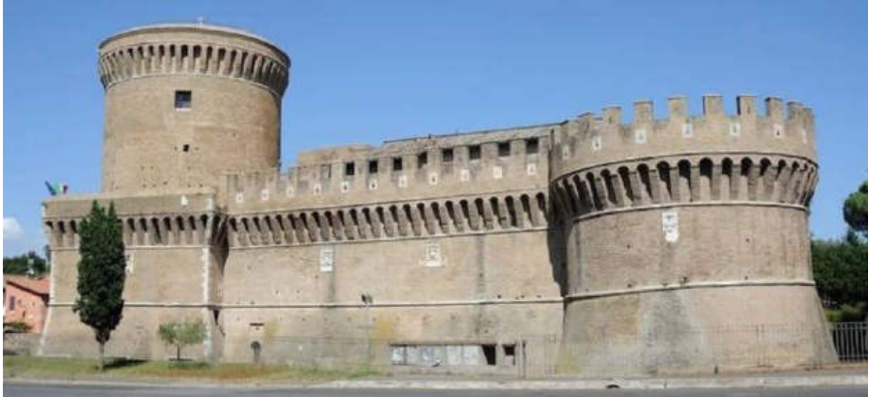
View of the east side of the Castello di Giulio II with the tower and southern roundel.
