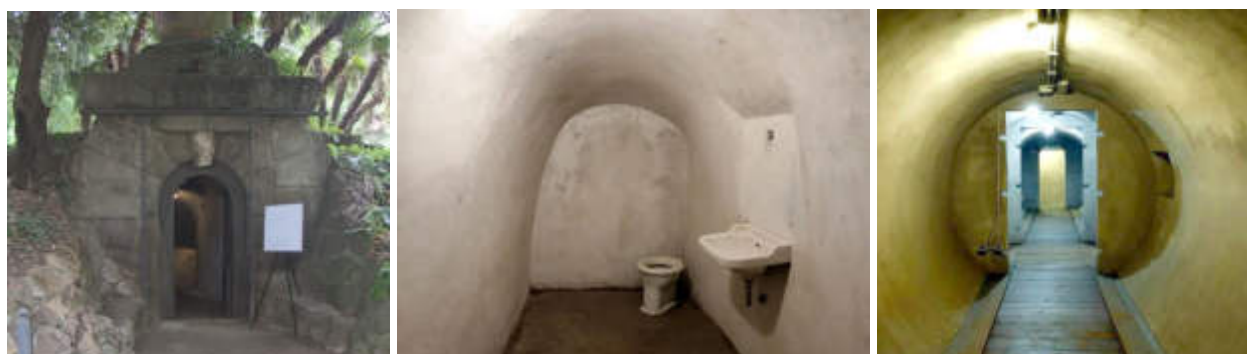
Bunker complex Villa Torlonia: entrance in the park, toilet corner, access tunnel.
