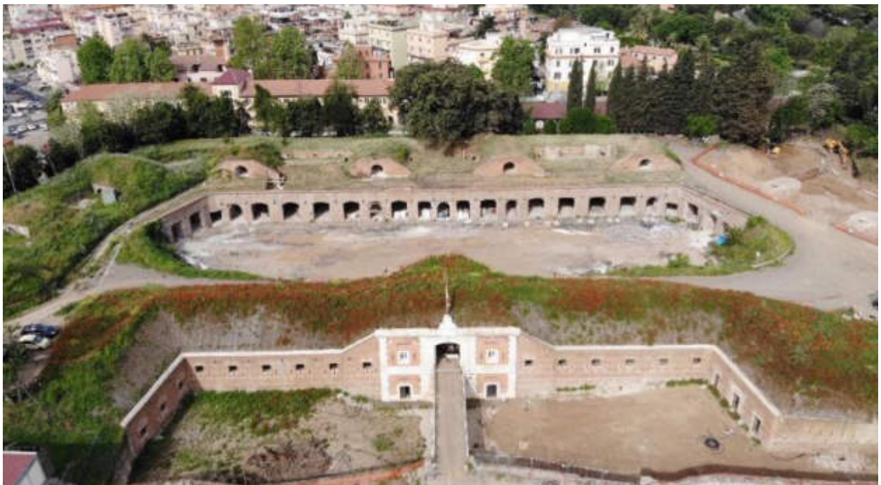
Aerial view of the restoration work at Forte Aurelia Antica.
