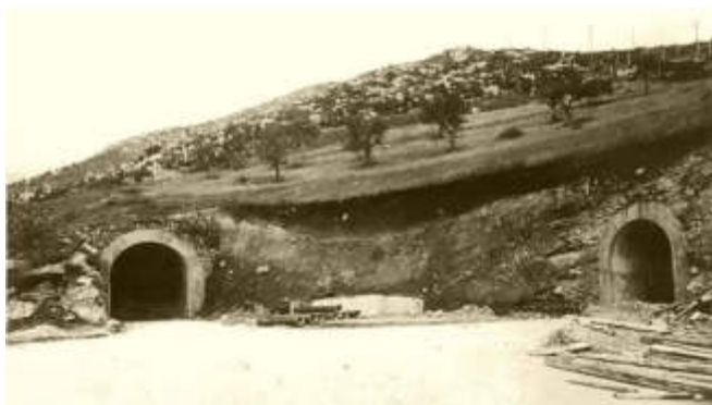
Tunnel entrances during construction 1939 ff.
