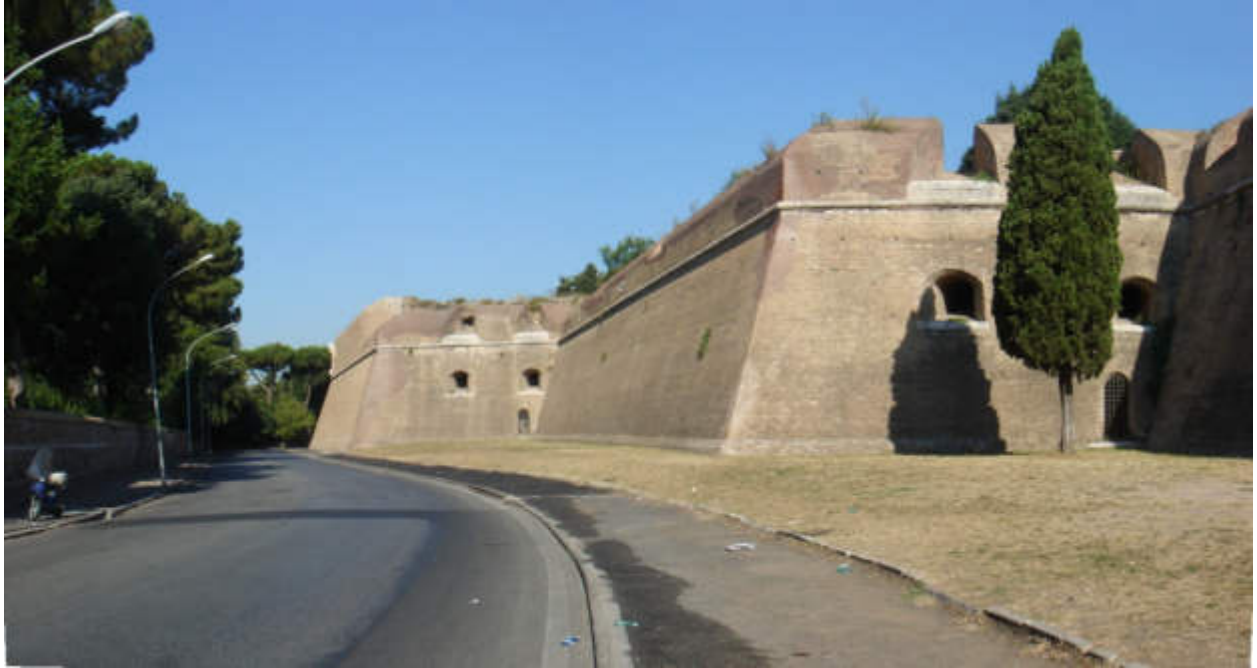
Sangallo-Bastion as part of the Aurelian Wall
