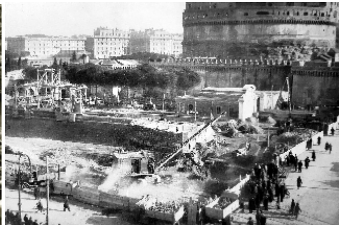
Restoration work on ditches and ramparts 1933
