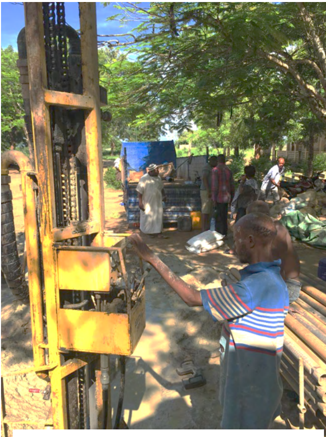
Drilling equipment arrives on site and the contractors begin to sink the borehole for the pipes
