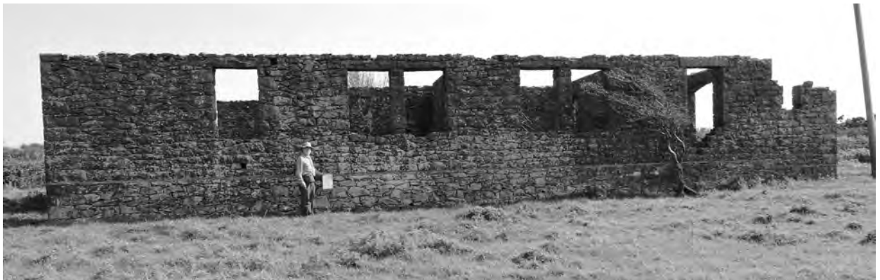
Partly constructed quarrymen's cottages on the site of model village
