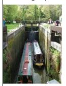
As you reach the main road you pass Widcombe Deep Lock (number 8/9). This was created when the canal was restored, and the road bridge constructed. It is 5.92m deep, making it Britain's second deepest lock.
