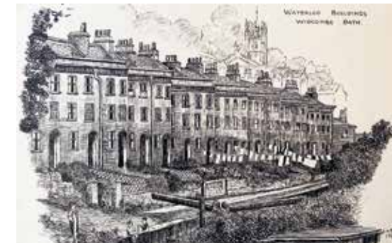
Waterloo Buildings recorded by S. Marks 1964 before demolition
